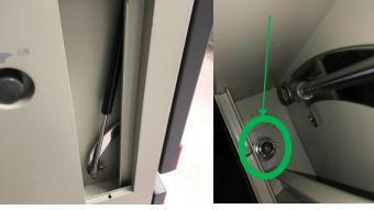
3. Use the spare service key (supplied with the unit) to open the back service panel, and remove the service panel.
